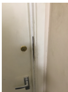
Damaged door frame
