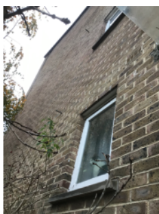
External walls of brick/mortar construction.
