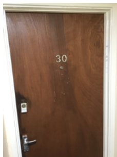
Replacement timber flat entrance door
