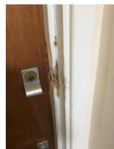
Damaged doorframe
