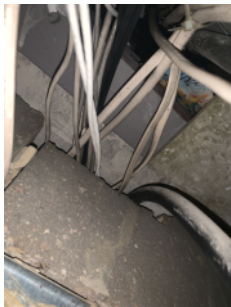
Example of cable penetrations with no fire stopping in riser cupboards.
