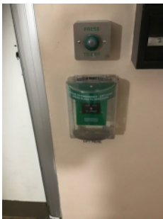
Door release, with additional emergency door release provided.
