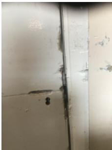
Severe damage to gas meter cupboard door.
