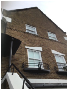
Brick and mortar external walls
