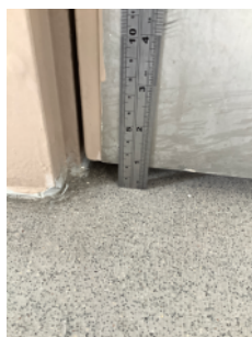
Threshold gap, 20mm, second floor lobby door
