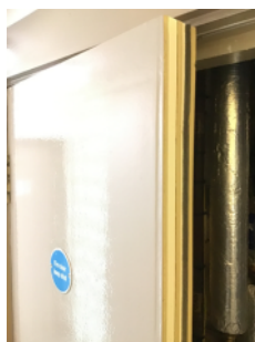
FD60S doors installed in risers.
