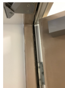
Intumescent strips and cold smoke seals on flat entrance doors
