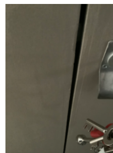
Excessive centre gap on riser door
