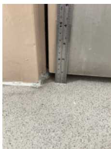
Threshold gap, 20mm, first floor lobby door
