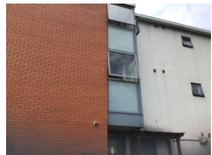
External walls, part brick, part rendered.
