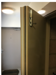
FD60S doors installed in risers
