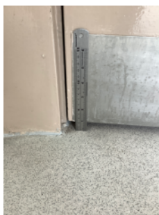
Lobby door threshold gap of 20mm
