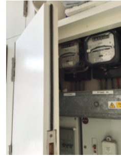
FD30S construction enclosing electrical installation
