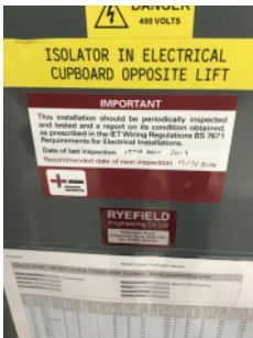
Valid test label on fixed installations.
