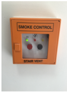
Smoke control override, showing status “ok”
