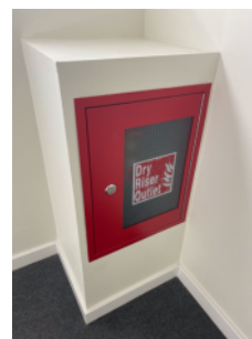
Dry riser outlets located within the staircase
