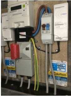
Repeater meters within risers.
