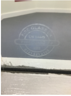
Acid etching, on staircase door glazing
