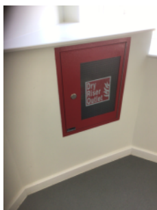
Dry riser outlets provided within the staircase
