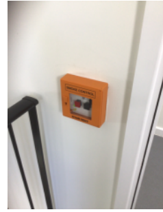
Manual smoke control device
