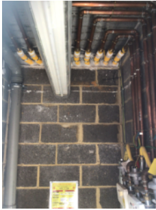
Fire stopping within the gas meter cupboard
