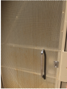
Vented door to gas meter cupboard
