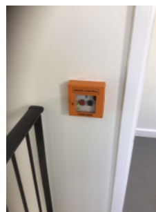
Manual smoke control device
