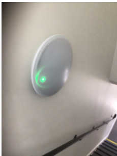
Maintained EL provided in common escape routes.
