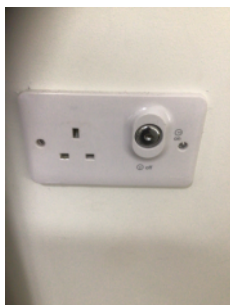
Key isolated electrical sockets are provided.
