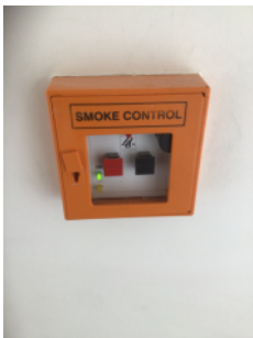
Manual smoke control device.
