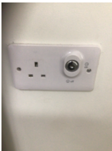
Key isolated electrical sockets are provided.
