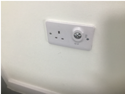
Electrical socket with isolating lock
