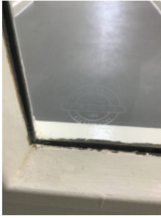
Acid etching, on staircase door glazing
