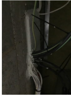
Example of fire stopping within riser cupboards.
