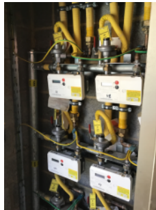
Gas installations in secured externally accessed enclosure
