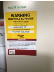
Evidence of testing of fixed electrical installations
