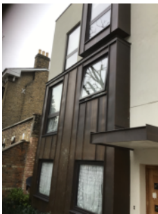
Metallic ring screen and front face of building and around window openings
