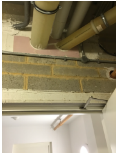
Fire stopping in basement
