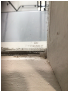
Acid etching on FR glazing installed in the staircase doors
