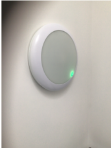
Maintained EL in the staircase
