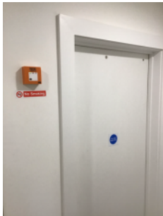
Wrong signs on smoke vent signs
