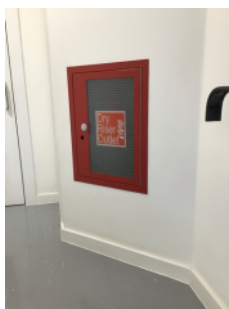
Dry riser outlet on each landing
