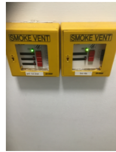
Smoke vent controls - ground floor.
