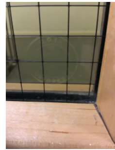
Acid etching on door glazing.
