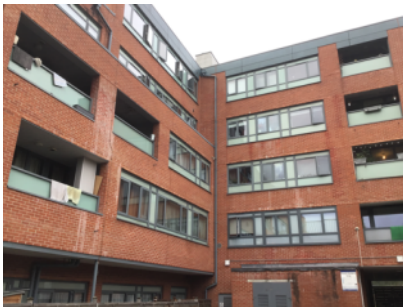
Brick/ mortar external walls with glazed panels
