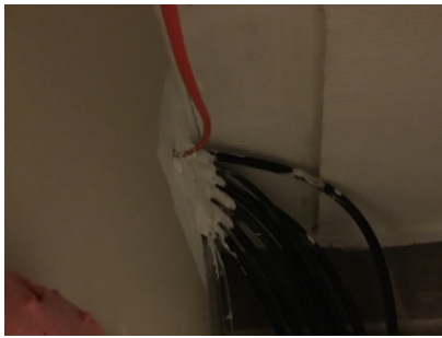
Example of fire stopping within riser cupboards
