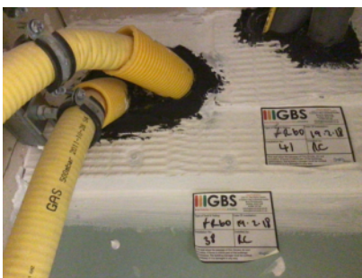
Evidence of fire stopping within riser cupboards conducted in 2018
