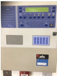
Main fire alarm panel
