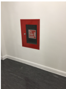
Dry riser outlet on each landing
