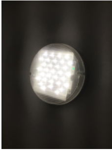
Maintained EL within the staircase
