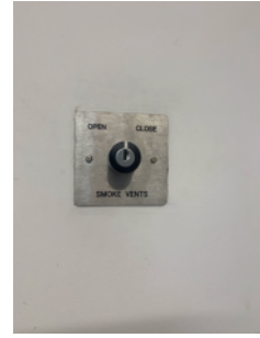
Manual smoke vent controls
