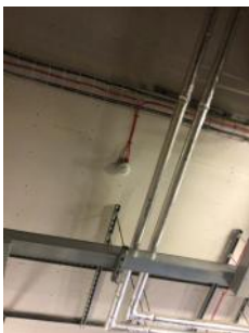
Part 1 heat detector in plant room
