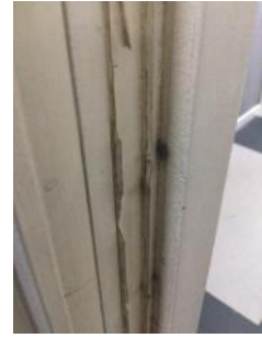
Damaged / worn neoprene smoke seals
