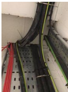
Fire batt requires sealing
