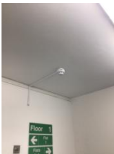
BS5839 Part 1 detection in staircase
