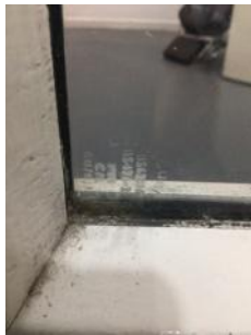
FR glazing etching on fire door vision panel
