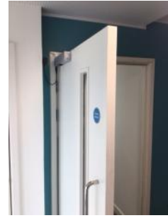
'Automatic Fire Door Keep Clear' signage is required
