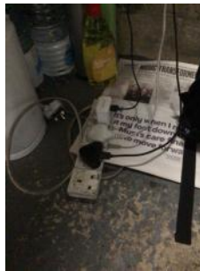
PAT testing required in Waking Watch office
