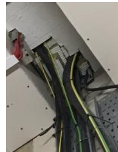
Poorly applied fire stopping in plant room / Waking Watch office
