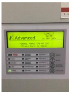
Main fire alarm panel showing a healthy status
