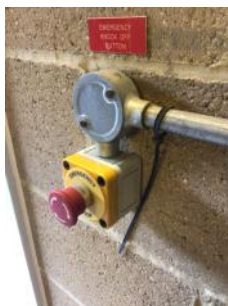
Emergency gas shut off in plant room
