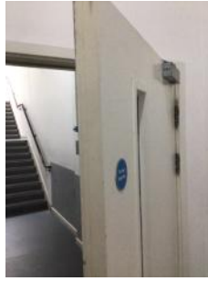
FD60S SC door to staircase
