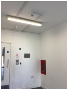
Normal lighting with motion sensor
