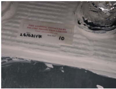
Example of fire stopping certification label - IMS Fire Protection Ltd 2017
