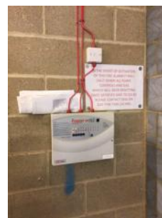
Fire alarm panel in plant room showing fault condition
