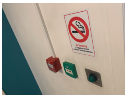
Manual call points located at each floor exit
