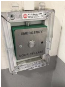
Emergency door release - main entrance/exit door
