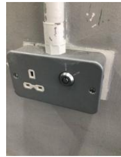
Key operated electrical socket - common area
