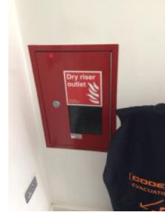
Dry riser outlets on all upper floors
