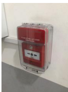
Manual call point by fire alarm panel
