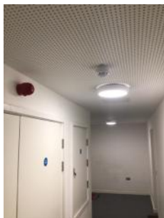
Smoke detector and sounder in common lobby
