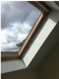
Window AOV appears defective
