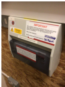
Evidence of testing of fixed electrical installations
