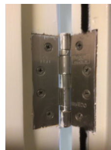
CE1121 marked fire rated door hinges fitted on electrical cupboard door
