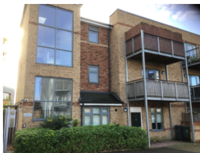
Brick/mortar external walls- front elevation
