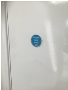
Keep locked shut signage on riser doors
