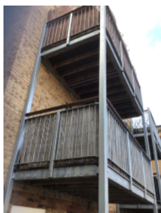
Steel framed balconies with timber deck
