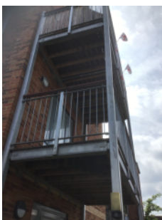
Construction of private balconies
