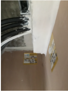
Evidence of Fire Stopping in risers cupboards
