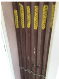
Gas pipe work in good condition, and correctly labelled in riser cupboards.
