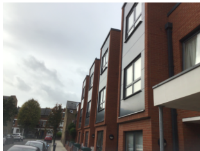
Brick/mortar external walls with an unidentified material window rainscreen
