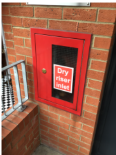
Dry riser inlet, adjacent main entrance door.
