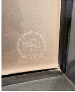
Acid etching of flat door glazing
