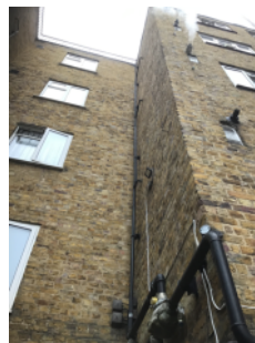
Original brick/mortar wall construction
