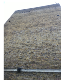
Original brick/mortar wall construction
