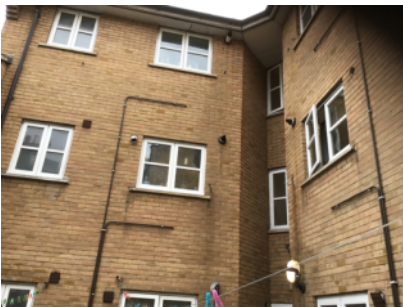
External walls - rear elevation
