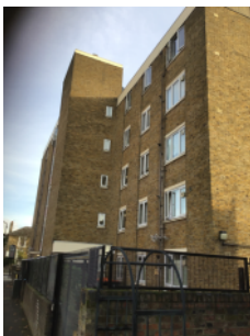
Brick/mortar external walls, side elevation
