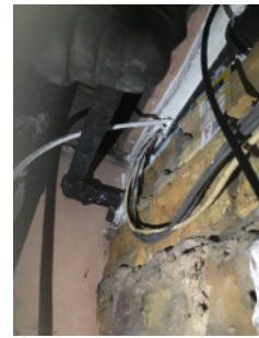
Evidence of recently installed fire stopping in risers
