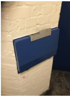
Refuse chutes in good condition
