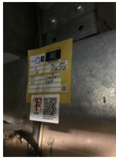
Evidence of recently installed fire stopping in risers
