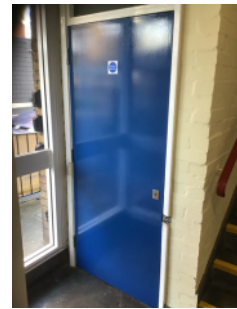
Basement door - the basement could not be accessed.
