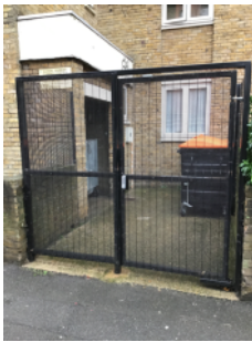
Secured bin chute at ground floor exterior level.
