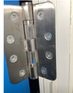
CE1121 fire rated door hinges fitted on staircase doors.
