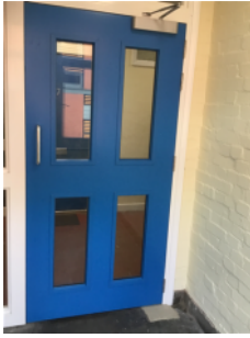
FD60S SC doors in staircase.
