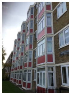
External walls- front elevation, with uPVC windows and wall panels
