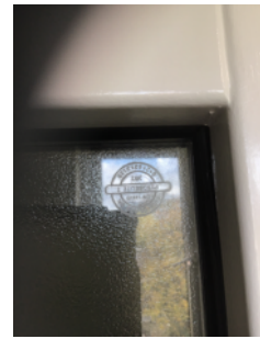
FR Glazing on flats windows and fanlights on corridors
