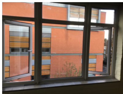
Openable windows in the staircase
