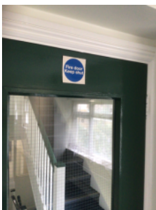
Fire door signage on self-closing fire doors.
