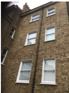
External walls-rear of the building.
