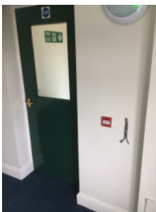
Manual call points are located at storey exits and the final exit.
