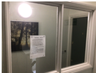
Georgian wired glazing in corridors.
