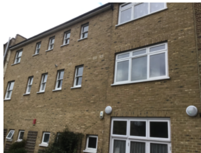
External walls-rear of the building.
