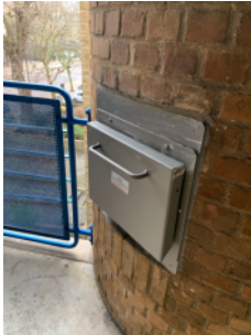
Rubbish chute hatches in good condition
