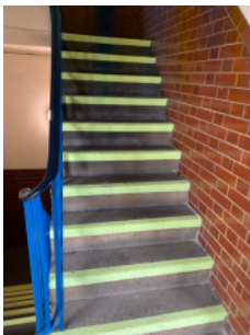
Stair nosings are of a contrasting colour to assist identification.
