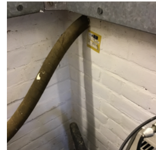
Version 3 - Evidence of fire stopping in lift motor room
