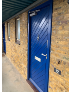
Example of flat entrance door with visible external self closing device
