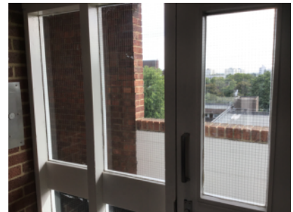
Georgian Wired glazing installed in the staircase partition.
