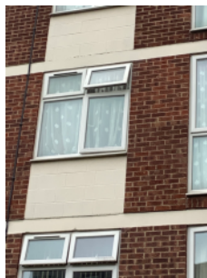
Close up - external walls, rear elevation
