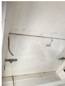
It was not possible to access the roof space
