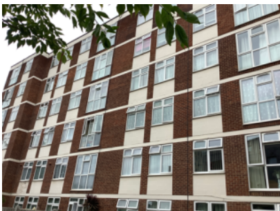
External walls, rear elevation
