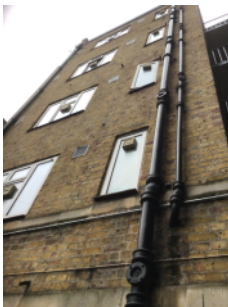
Original brick/mortar walls.
