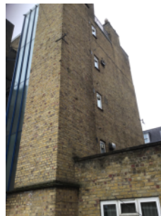
Original brick/mortar walls
