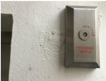
Firefighters switch to lift (not tested during this inspection)
