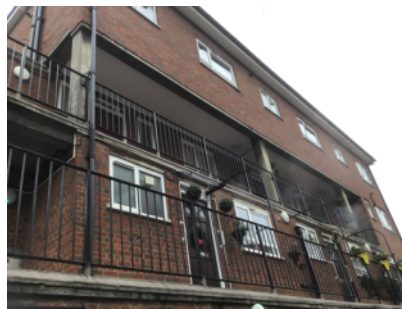
Brick/mortar external walls
