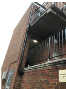
Brick/mortar external walls
