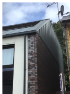
Photograph showing shape of roof
