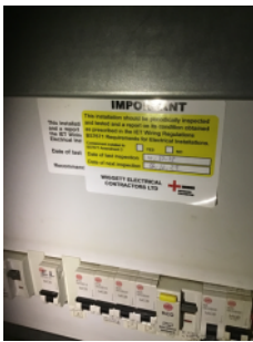
Evidence of testing of fixed electrical installations
