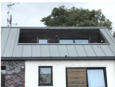
A timber cladding system surrounding 2nd floor balconies, front elevation
