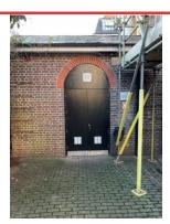
REAR DOOR STUCK CANNOT OPEN FULLY WOOD EXPANSION Assigned To Delta Raise wo REP-044793
