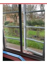
**CLOSE TO DOOR 4 AND 6 STAIRWELL MISSING LEVER**
