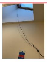
**CABLE IS USED TO OPEN WINDOW**
